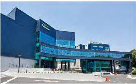
HMR wet noodle plant
